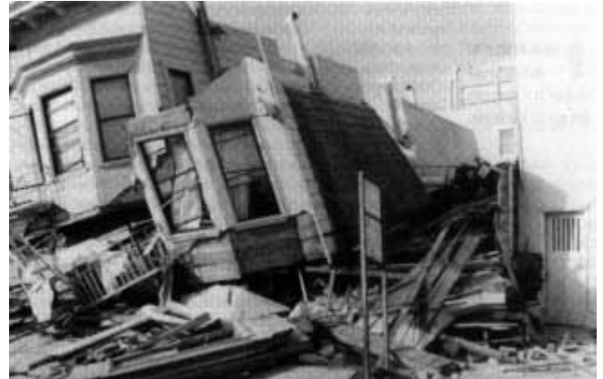
Figure 21-1 Loss occurs with the destruction of property. Think of the many losses that are experienced by the family whose home was destroyed in an earthquake.
