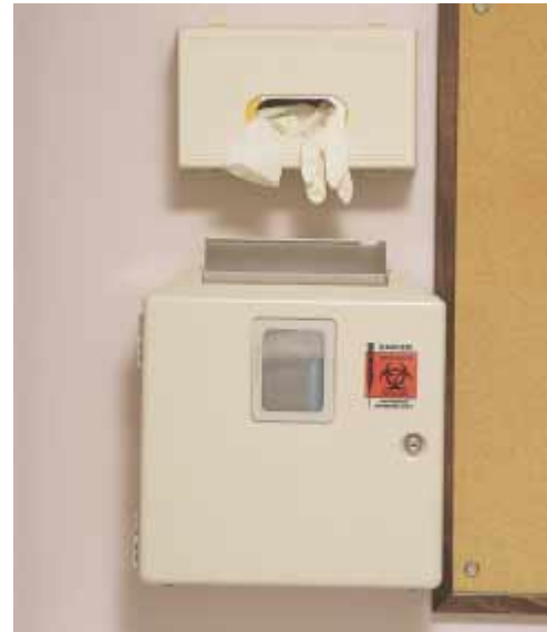
Figure 31-23 Sharps Disposal and Infectious Waste Containers
